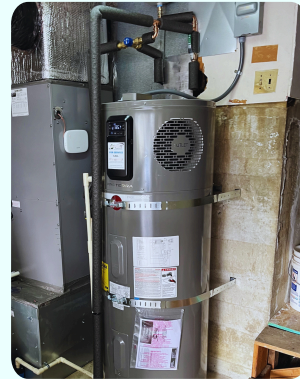
Davis Residence with Upgraded Circuit Splitter and HPWH
