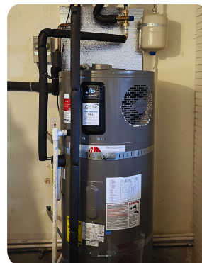
Davis Residence with Upgraded Circuit Splitter and HPWH
