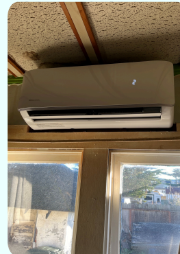
Kim Residence with Upgraded Induction Range and Ductless Mini Split
