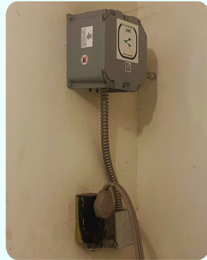
Davis Residence with Upgraded Circuit Splitter and HPWH
